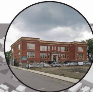
INSPECTIONAL SERVICES DEPARTMENT BUILDING
